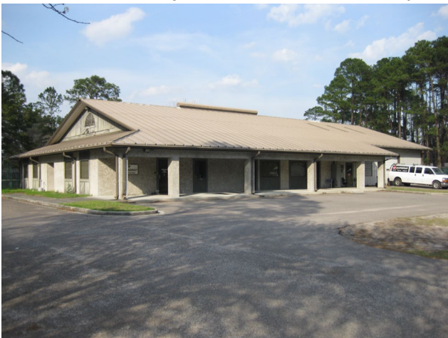
E: Office building on subject
